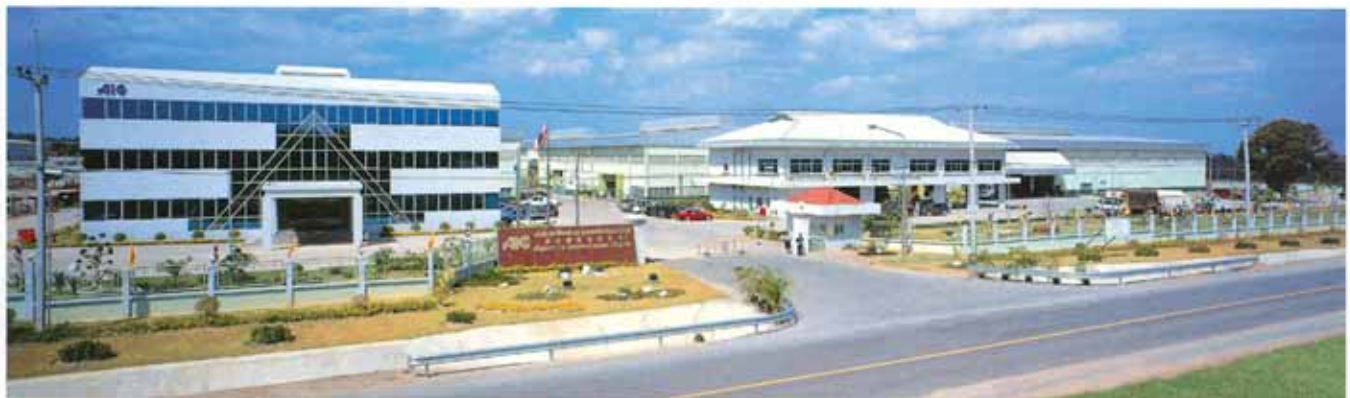
AEROFLEX INTERNATIONAL CO., LTD. HEAD OFFICE & FACTORY, RAYONG, THAILAND.
